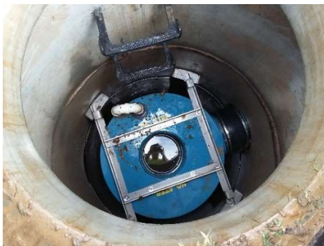
MAINTAINED DETENTION STRUCTURE
