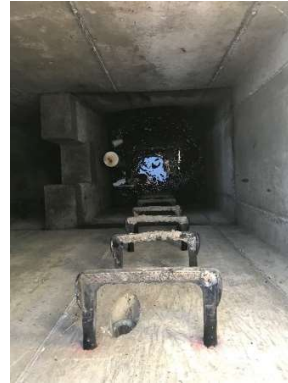
DETENTION PIPE NOT MAINTAINED
