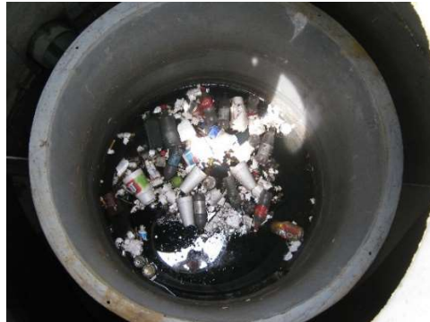
DETENTION STRUCTURE NOT MAINTAINED
