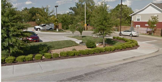
MAINTAINED BIORETENTION BASIN
