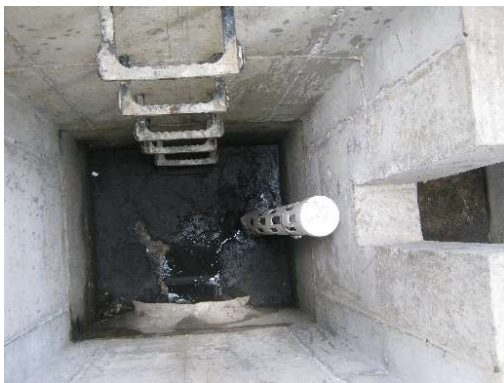
MAINTAINED DETENTION PIPE
