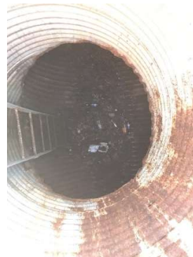
DETENTION PIPE NOT MAINTAINED
